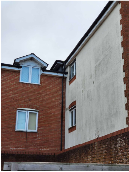
Exterior Structure (The Building)
